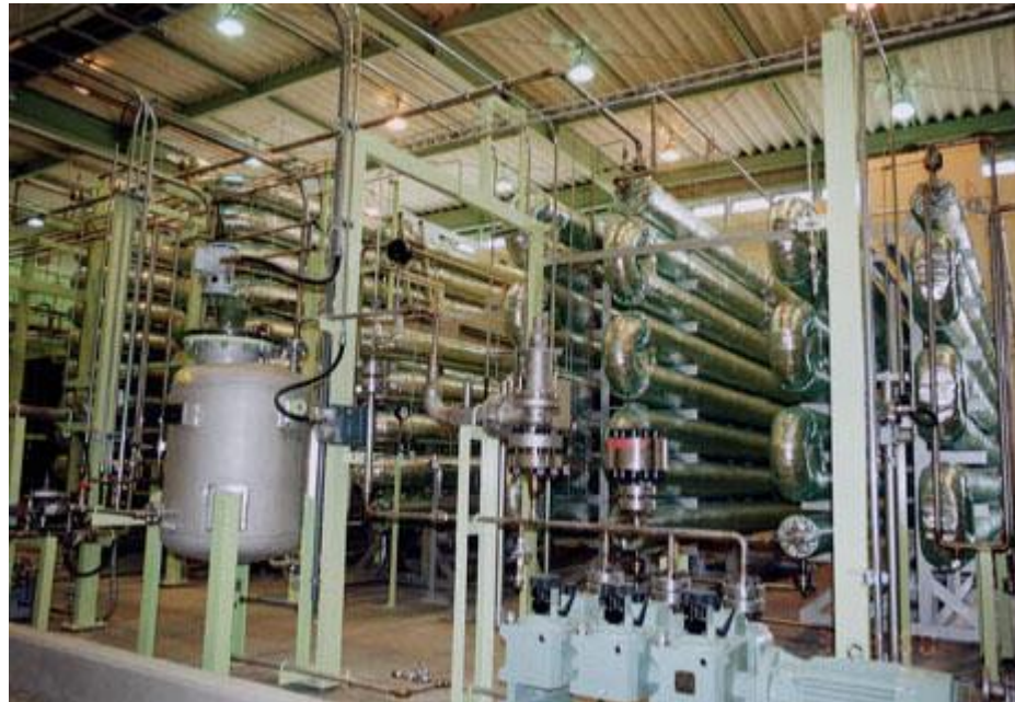
Shinko Pantec's pilot plant , Japán, 1.1 m 3 /h
