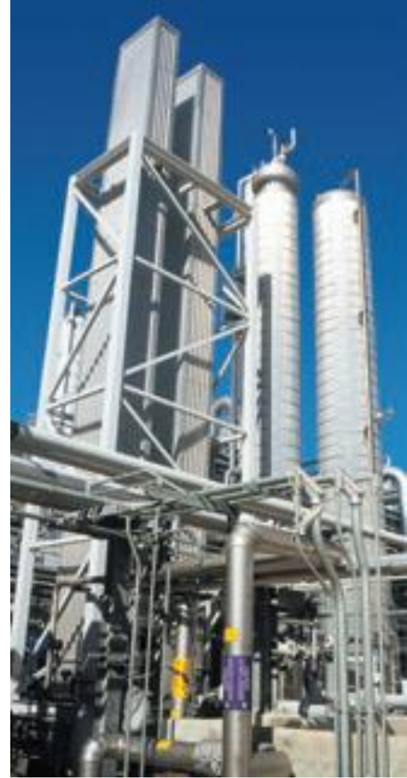
BASF ethylene facility, Port Arthur, Texas.
